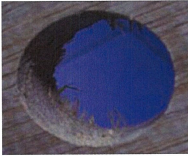
Figure 12 Tear-outs from boring test
