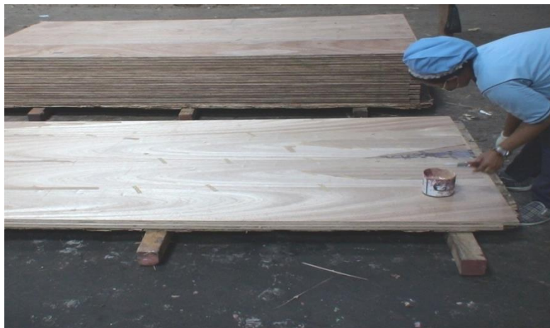
Figure 9. Plywood putty process.
