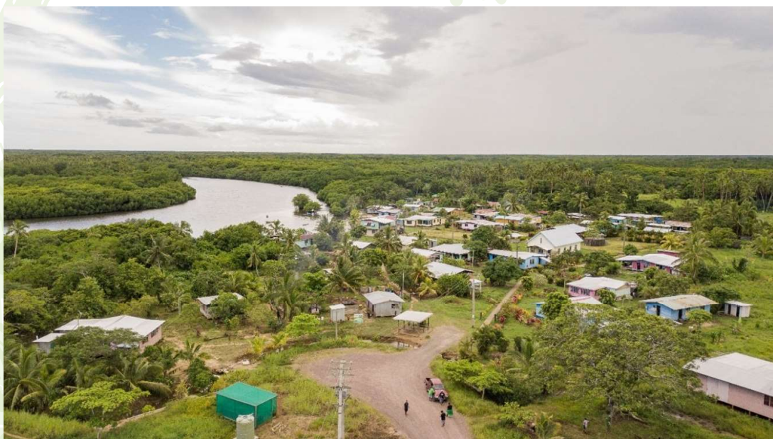
Figure 13: Mangroves are often cleared to accommodate new infrastructure and development constructions, Rewa delta, Viti Levu
