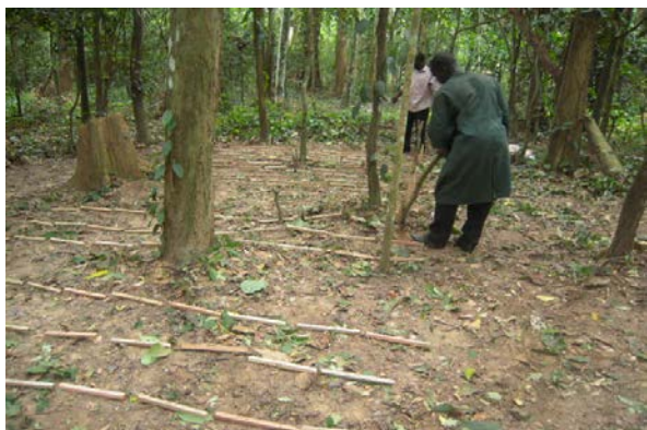
Figure 7.1: Site preparing for graveyard test
