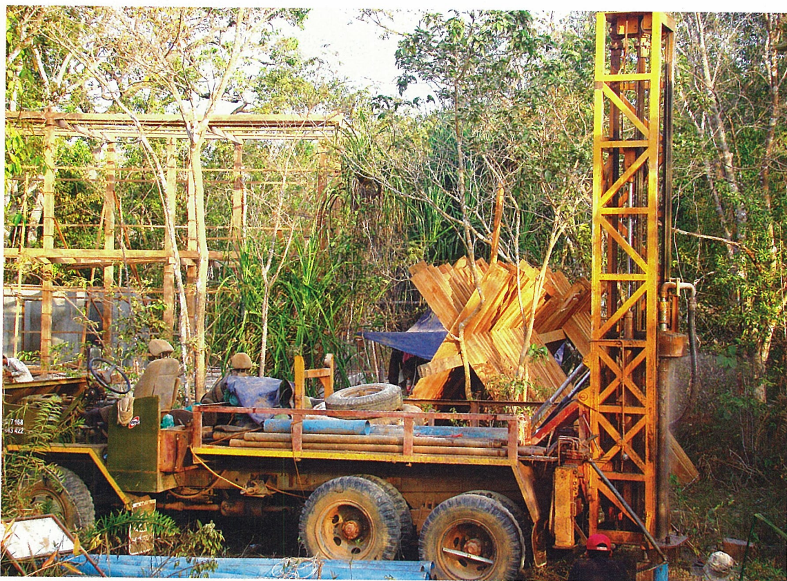
Drilling a pumping well for Ranger Outpost at Mombei in the Preah Vihear Protected Forest near the Cambodia – Lao – Thai Tri-Border
