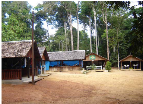
Output 1.2 – Camp facilities upgraded
