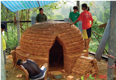
Bamboo Charcoal Kiln Construction
