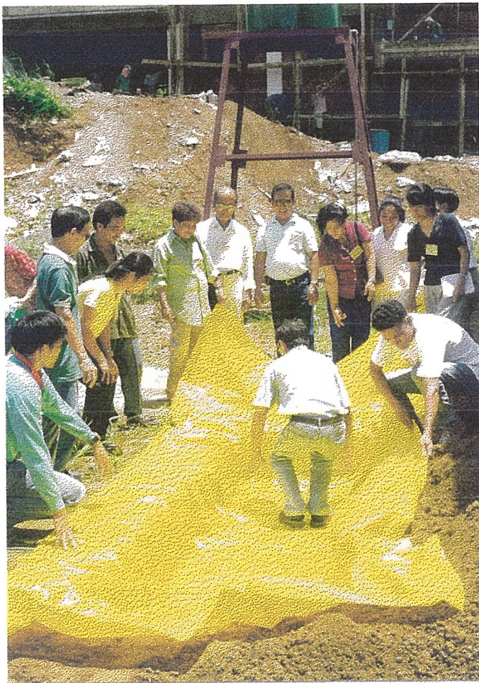
The participants laying the plastic sheet in the Trench.
