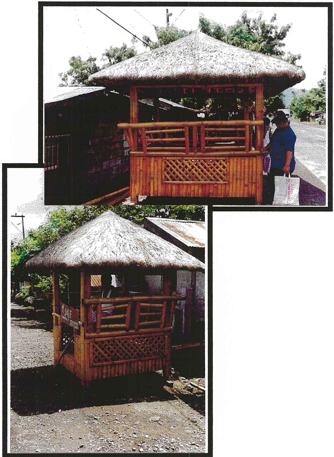
Bamboo house, a common sight along roads going to Lucena City, Quezon province.
