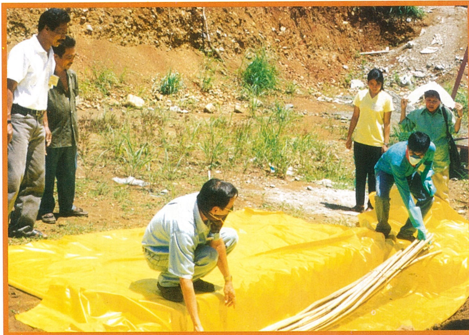
Placing rattan canes in the plastic lined trench.
