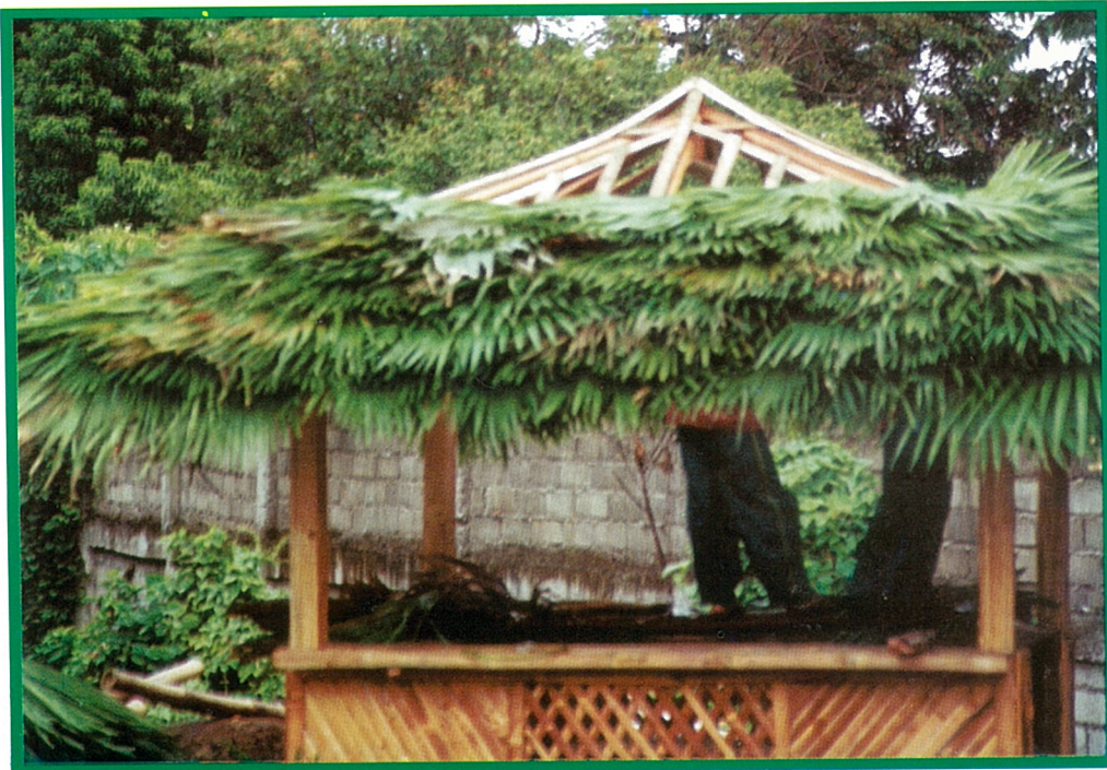
8B. Leaves of Livistona being used as roofing material for bamboo rest house.
