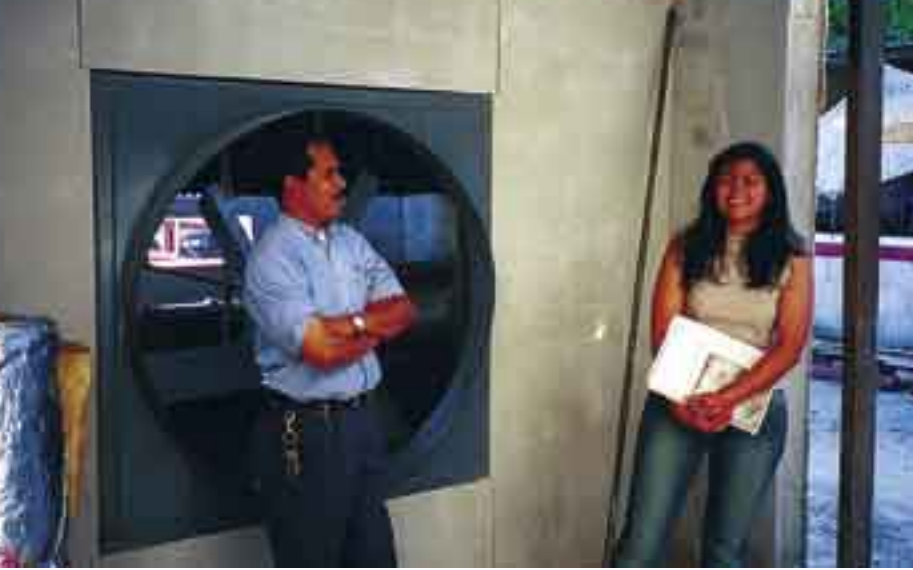
Sunny perspective: ESNACIFOR's Heidi Vides chats with a member of the San Pedro Sula cooperative next to a solar drying kiln under construction. Photo: J. Peltonen
