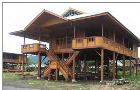
Packed with cempaka: A traditional Minahasa house made predominantly of cempaka wood. Photo: Muh. Farid/MEFRDI
