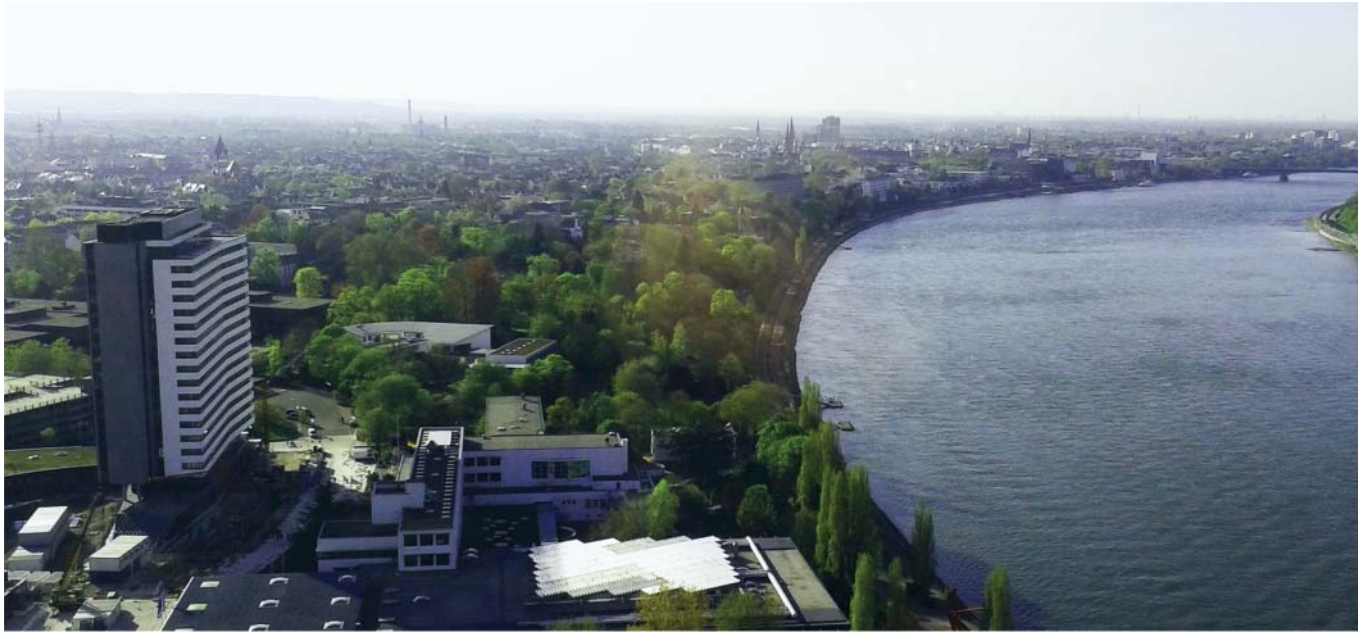
The city of Bonn in Germany recognises “blue-green” corridors in its planning measures (Photo: Nidbi Nagabhatla)
