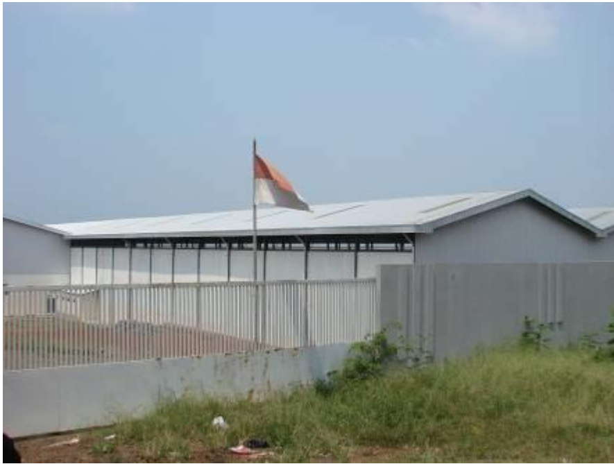
Newly constructed plywood mill (PT. J-Cool) in west Java
