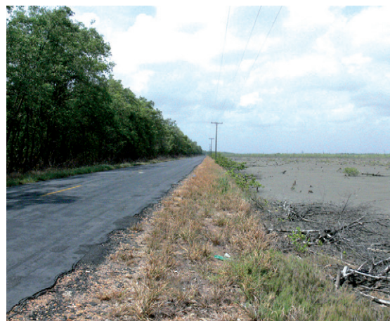
The bare ground on the landward margin of this road in Brazil has lost all its mangroves as a result of changes in water flow. Photo: S. Baba
