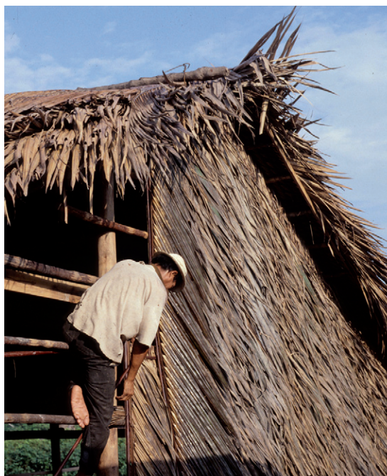
The leaves of Nypa palms are widely used for thatching, such as on this house in Viet Nam. Photo: S. Baba
