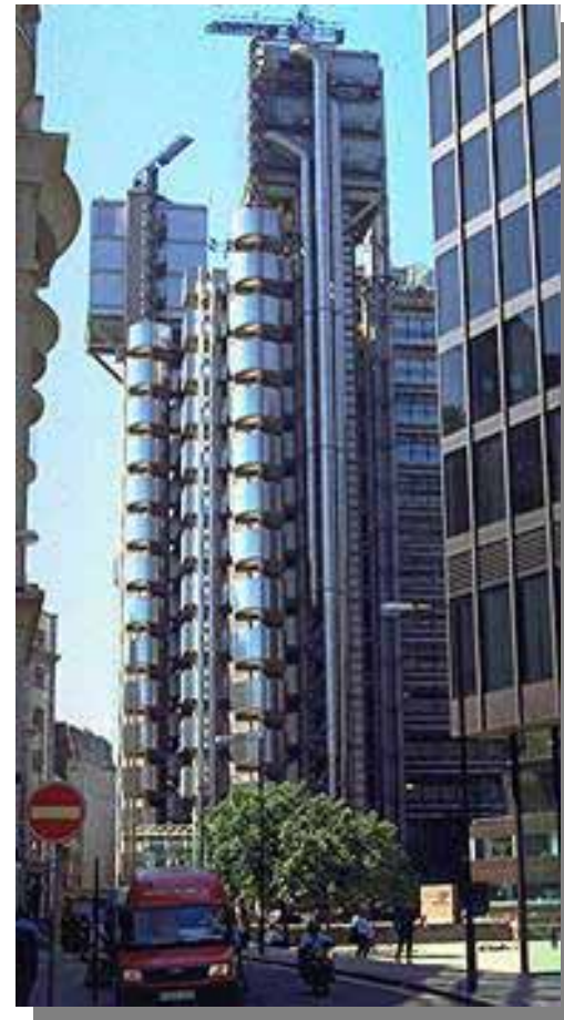
Lloyd's of London building
