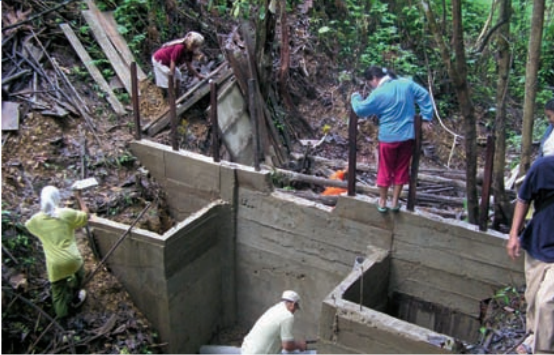
Concrete action: Longhouse members work with project staff to construct a valley pond. Photo: S. Lanjang
