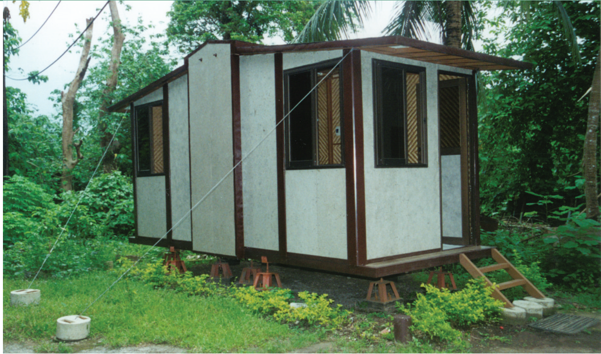
Home sweet home—the fully erected F-house. Note the tension cables (or tie-down straps) attached to ground anchors. Photo: FPRDI
