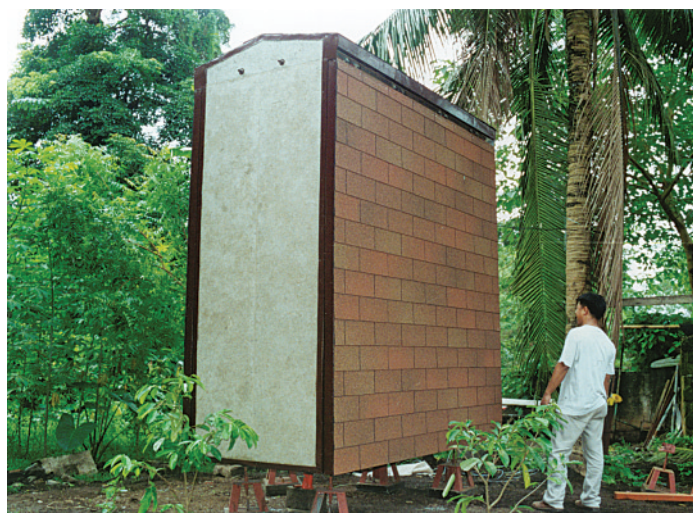
The F-house arrives in its case ready for 'unfolding'. Photo: FPRDI
