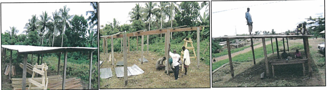
Figure 4: Lumber drying sheds in construction at two communities
