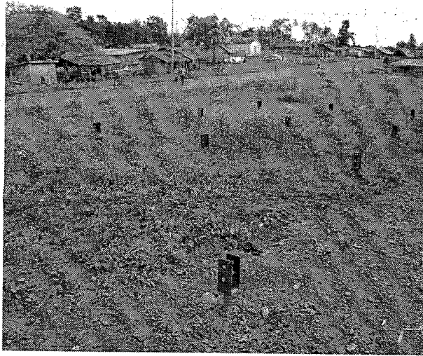
Plate 12: The U-plates to hold the poles in position for shed construction at Dominase
