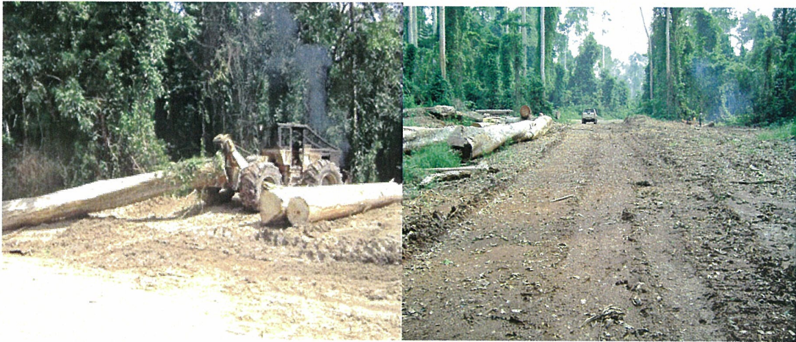
Figure 14: Disturbed areas due to heavy duty machinery logging
