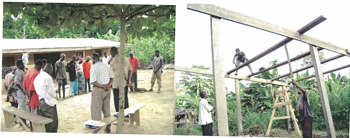
Figure 16: Local community participation for the construction of lumber drying shed
