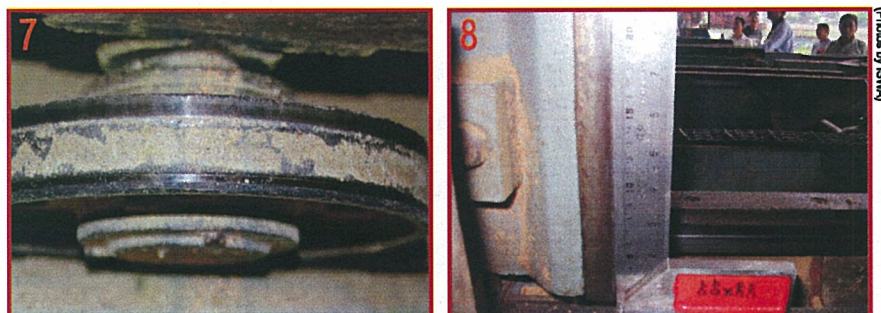
Figures 7-8. Wheel covered by sawdust (7); log skid bed and kneenot not perpendicular (8)
