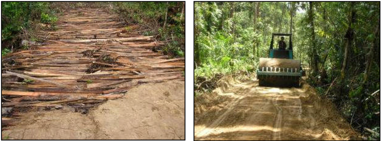
Figure 7.2 Redger wood used as the middle layer and sand cover as the top layer in the forest road construction
