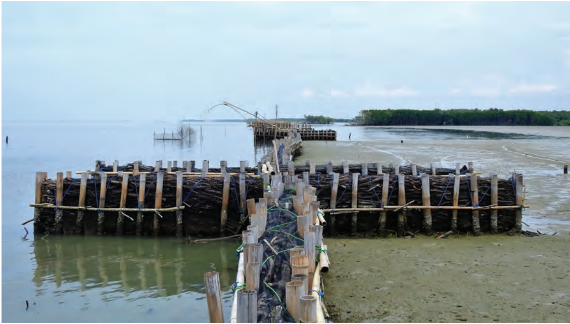
Holey wall: The aim of this porous sediment trap built by the Building with Nature Project in Demak, Indonesia, is to create suitable habitat for natural mangrove regeneration. Photo: Yus Rusila Noor
