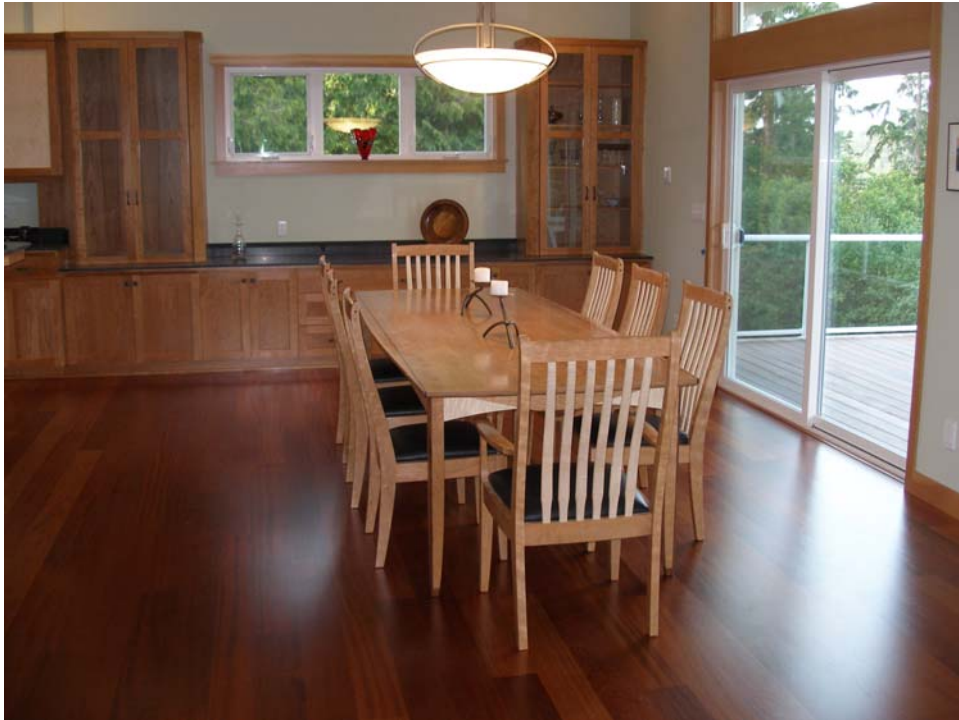
Px (a) Residential – Jatobá engineered wood floor with maple dining table (courtesy of Bill Altman)
