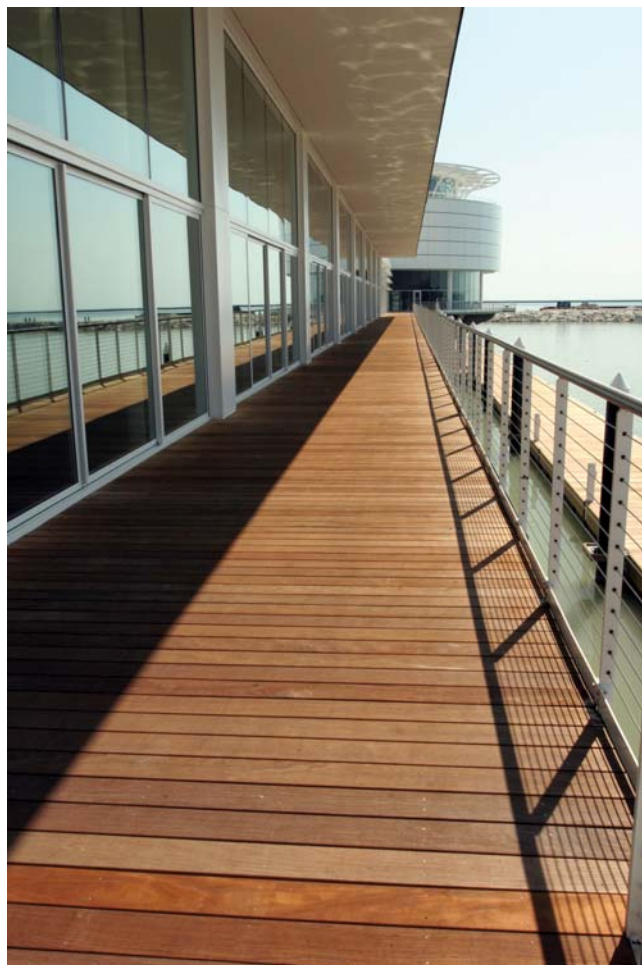
Px (j) Ipé decking on commercial project (Courtesy of IWPA)
